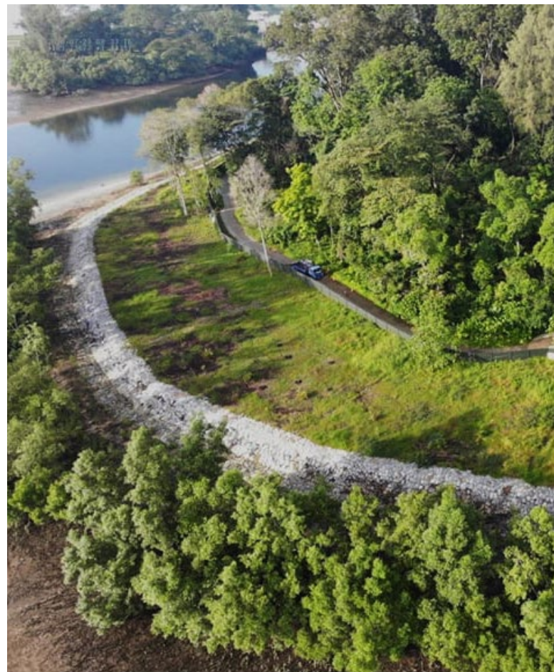
The National Parks Board of Singapore employs nature-based solutions for coastal resilience. A 400 m low rock revetment was erected to reduce wave energy and encourage accumulation of sediments at Kranji Coastal Nature Park. Photo: NParks.
